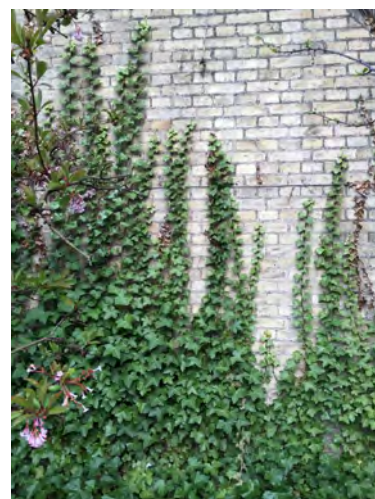
Begrønning af facade
